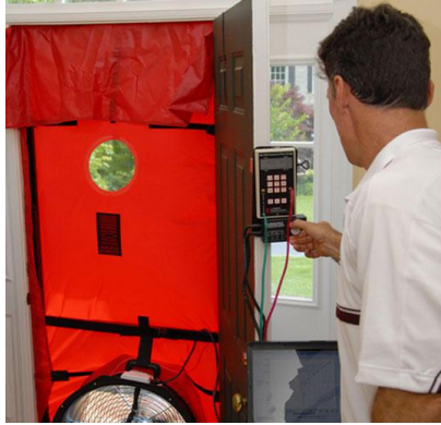
Photo Caption Ardently Green inspectors (certified by the Building Performance Institute) perform a “blower door” test, through which they can determine with infrared cameras where air is leaking between walls and floors.
